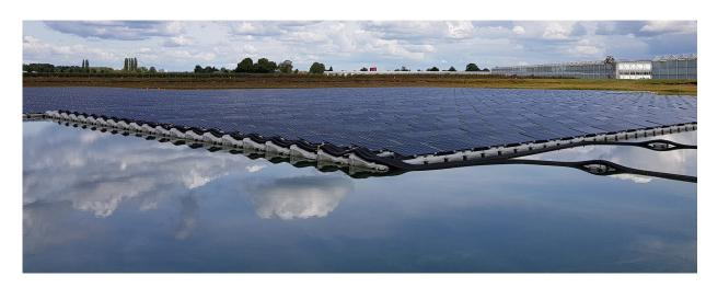
Located in a Netherlands irrigation water basin, the 1.845MW Lingewaard Floating Solar Park took an expanse of water and, in conjunction with SolarEdge, turned it into a green energy power source. Installed by Tenten Solar, the field produced 1 million kWh of energy from 6,150 panels, barely five months after installation on 31 August 2018.
