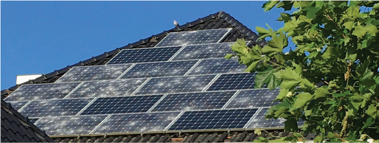
Photo by HD-Solar — The Netherlands
