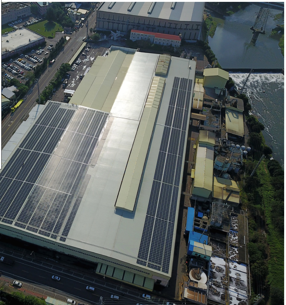
Solar production as viewed in the SolarEdge monitoring platform
