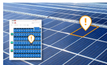
Pinpointed system alerts at the module level
