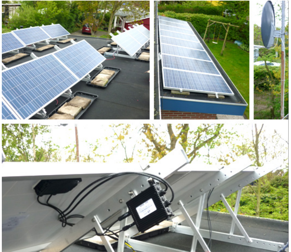
Photo: The photo shows the Centrotec test site in Ouddorp, Netherlands with two test systems used for a comparative case study between a regular inverter and SolarEdge.
