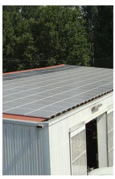
prevent power loss from mismatch between modules. Even if each module in a string had completely different electric parameters, they would still continue operating at their individual maximum output. Overcoming the mismatch between the modules allows the SolarEdge system to harvest more energy from the Tarascon installation than would a traditional inverter system. This advantage is very likely to increase over the next few years, as modules age and mismatch between them grows.
