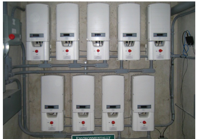
Figure 3: The SolarEdge inverters in the Donkers' utility room. Photo by Sashaan Solar
