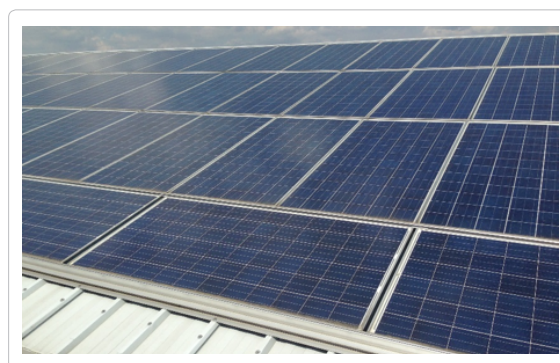
Figure 3: Photograph of string 15.2 does not reveal an apparent source for the mismatch between modules in the string
