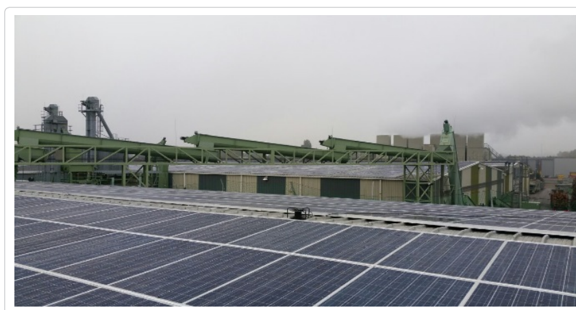
Figure 6: Trucks unloading dusty raw materials and smoke coming out of the Plospan chimneys generate soiling mismatch
