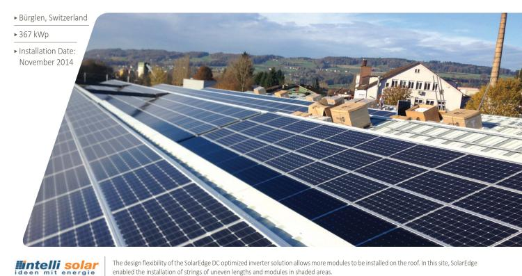
The design flexibility of the SolarEdge DC optimized inverter solution allows more modules to be installed on the roof. In this site, SolarEdge enabled the installation of strings of uneven lengths and modules in shaded areas.
