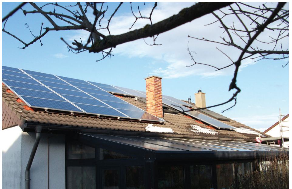
The photo shows how the SolarEdge system allowed Mr. Schneider to install modules close to the chimney without risking disproportional energy losses.
