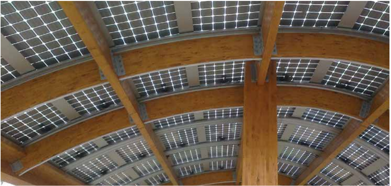
The Netherlands, 3MW 39 Electric Car Charging Stations
