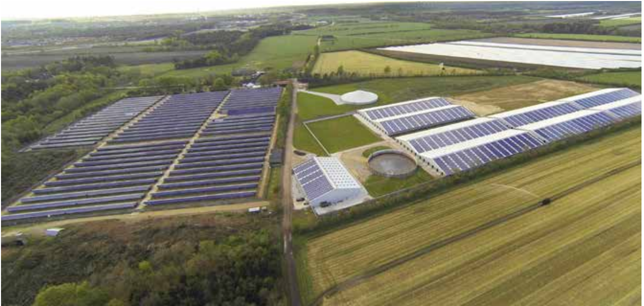
Denmark, 2MW Ground and roof mounted
