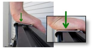
For North-America - Installation of the Zep Compatible SolarEdge power optimizers create automatic ground-bond connection with Zep Compatible modules, eliminating the need for any additional bonding hardware. The power optimizers can be installed on either the long edge or short edge of the module.
