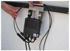
**4** Firmly press the bracket with your palm to install
