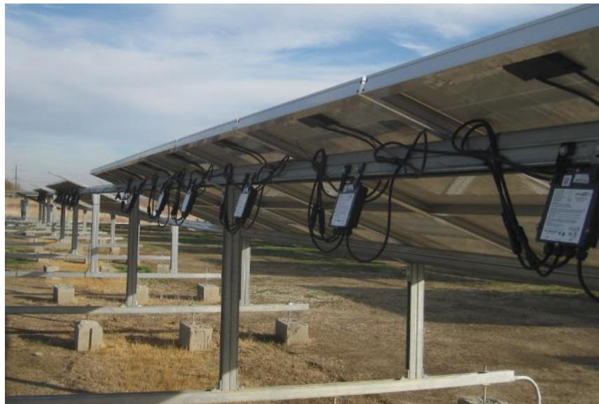
Figure 9-12 Test array with SolarEdge Optimizers Rack Mounted
