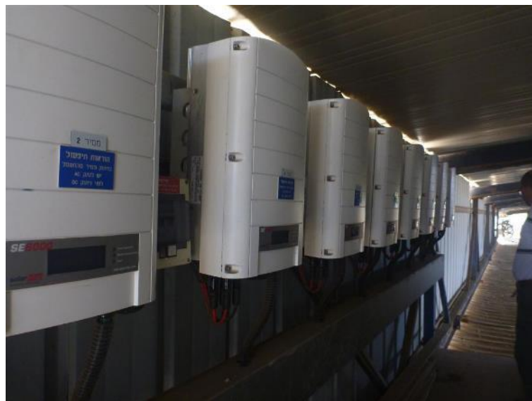
Figure 9-3 Solar Edge inverters at Green Tops Site
