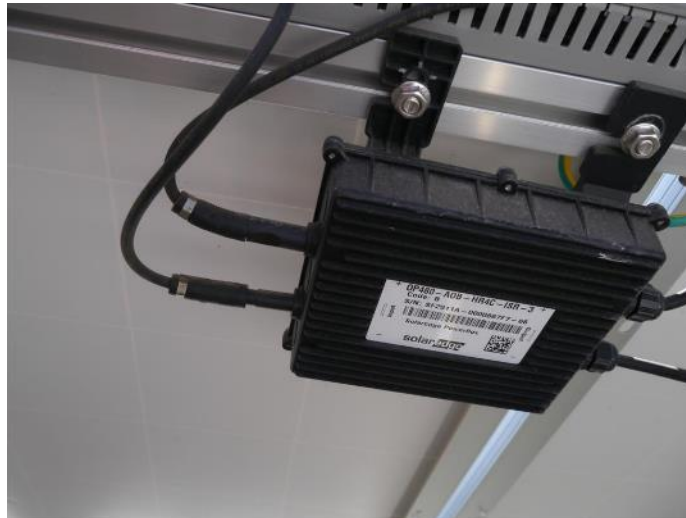
Figure 9-7 SolarEdge Power Optimizer at Dugma Site
