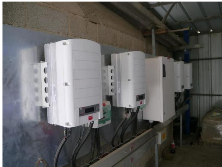
Figure 9-8 Solar Edge Inverters at Dugma Site
