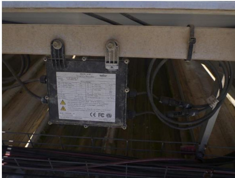
Figure 9-2 Early Generation SolarEdge Power Optimizer at Green Tops Site
