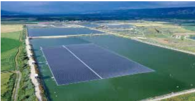
7.1 MW, Floating PV plant, Israel
