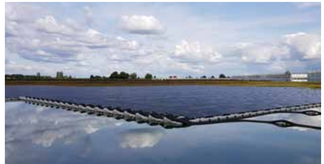
2 MW, Lingewaard Floating Solar Park, The Netherlands
