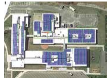
Project design validation prior to installation
