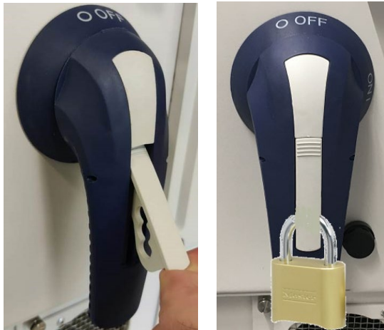
DCD switch safety padlock
