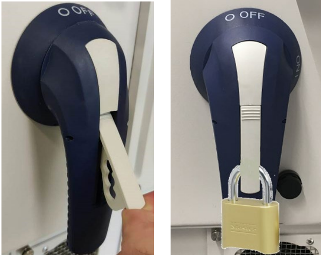
DC ON/OFF switch safety padlock
