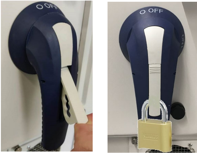
DCD switch safety padlock
