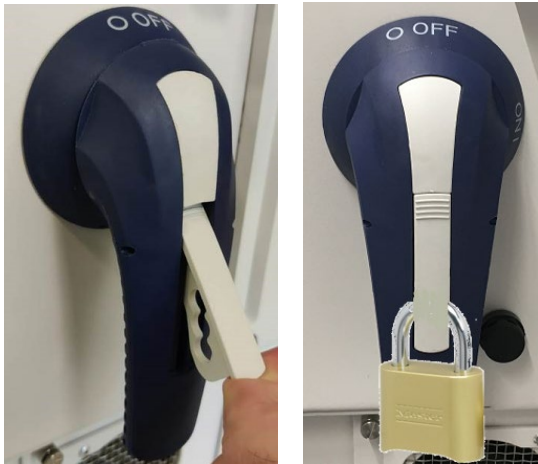
DCD switch safety padlock
