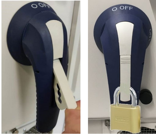
DC ON/OFF switch safety padlock
