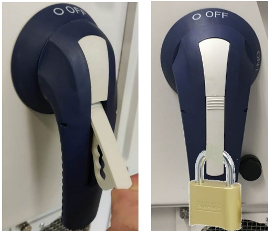
DCD switch safety padlock
