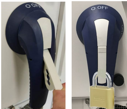
DC ON/OFF switch safety padlock
