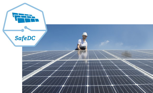
Figure 2: Touch-safe voltage levels with SafeDC™
