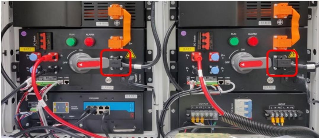
2. Reconnect the black cables at the top of the battery strings on both sides of the battery cabinet, as shown below.
