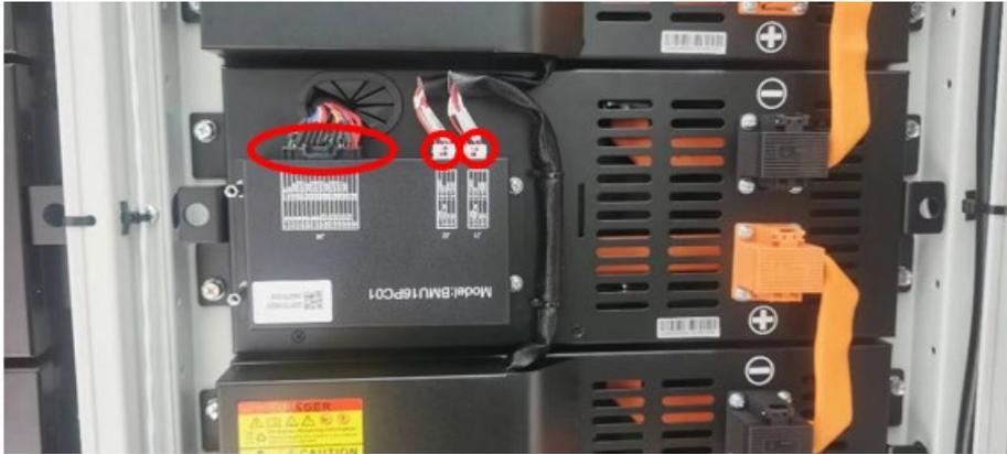
2. While pressing the tab, use a screwdriver to gently lift the connectors out.
