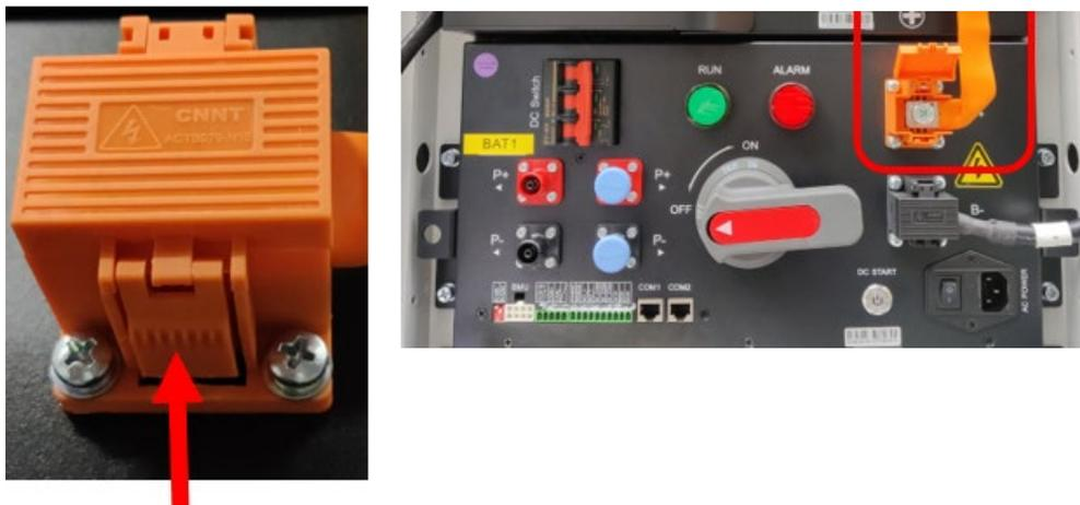
2. Use a 13mm socket and a wrench to remove the bolt securing the soft copper cable.
