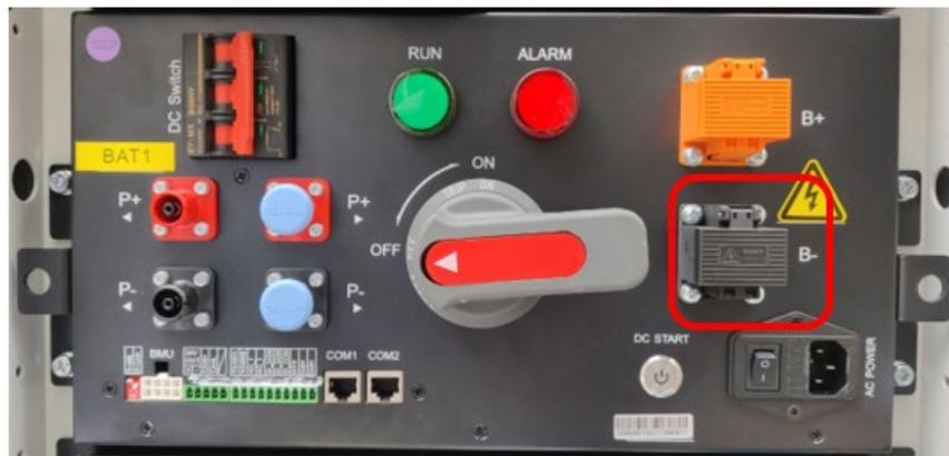
5. Use insulating tape to wrap the metal terminal of the black DC cable.
