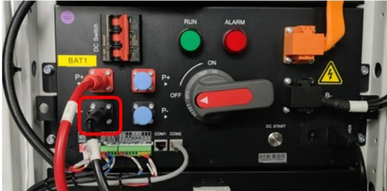
2. Plug the gray network cable into its connector.
