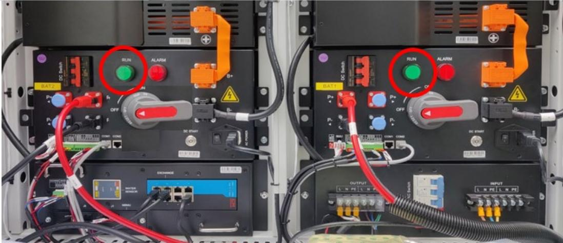
6. Ensure that the inverter indicator lights are OFF.
