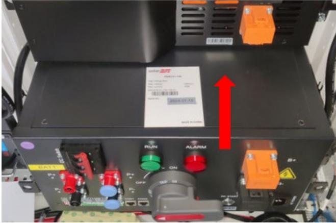
2. Using a 10mm socket and a wrench, fasten the 4 M6x16 bolts to a torque of 4.5N·m.
