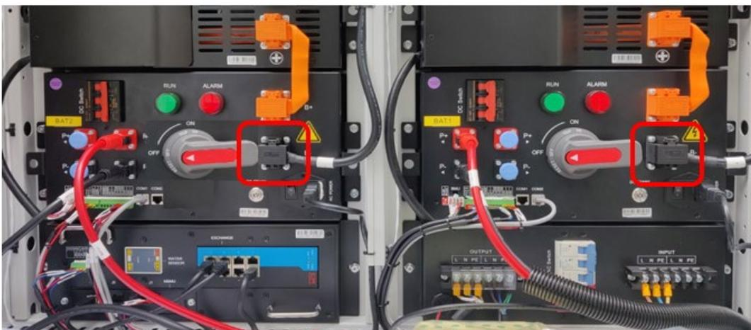
2. Reconnect the black cables at the top of the battery strings on both sides of the battery
