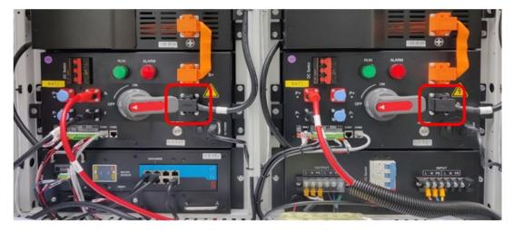
2. Reconnect the black cables at the top of the battery strings on both sides of the battery cabinet, as shown below.
