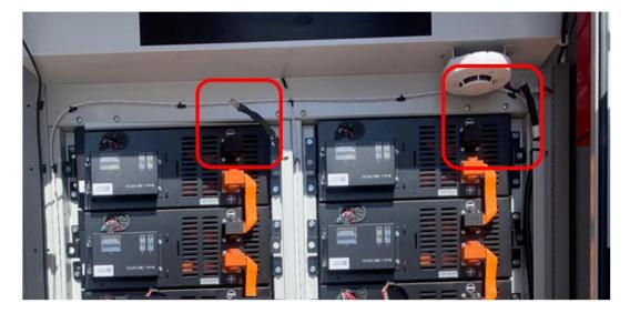
8. Disconnect the black cables from the bottom of the battery strings on both sides of the battery cabinet.
