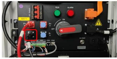
6. Plug the gray network cable into its connector.
