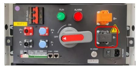
14. Use insulating tape to wrap the metal terminal of the black DC cable.
