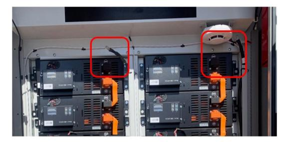
7. Disconnect the black cables from the bottom of the battery strings on both sides of the battery cabinet.
