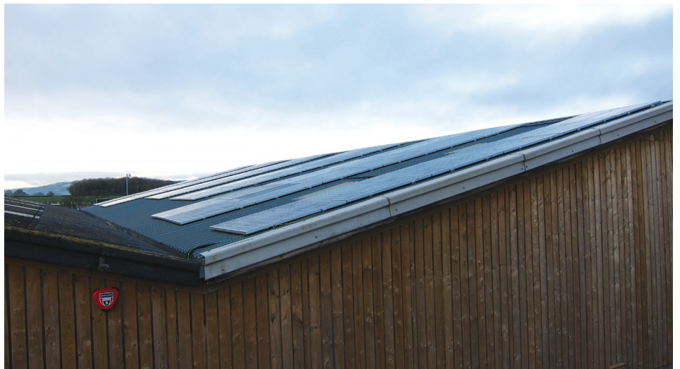
No energy losses occurring from partial shading. Installation in partially shaded area increases roof utilization
