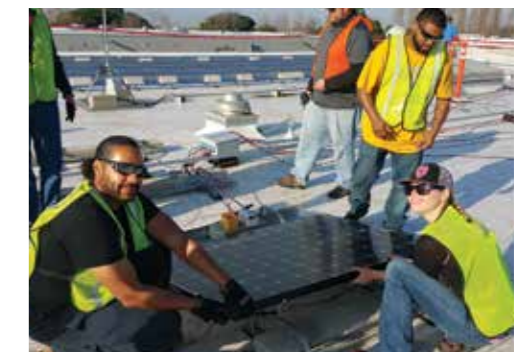
Teamwork to take this roof solar
