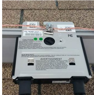
Figure 4: Grounding lug
