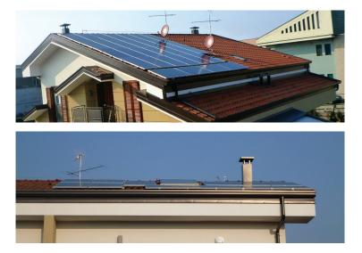
Despite the roof having two asymmetrical and opposite-facing facets, this system only has one 42-module string and is still able to maximize power from each individual module thanks to the SolarEdge module-level optimizers.
