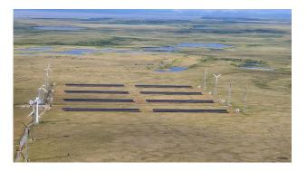
As part of the project, KEA decommissioned eight of their aging 66kW wind turbines and had the same power rating installed in the SolarEdge inverters. The SolarEdge power optimizers/inverters and LG bifacial panels were specifically chosen to maximize the energy yeild and for higher system uptime and low O&M costs.
