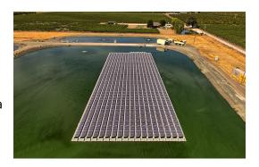
This included a 252 kW design, using Canadian Solar modules and SolarEdge power optimizers/inverters. The solution would cover the plant's annual kWh usage, and projected annual electricity savings of \$90,000, which would grow over time as PG&E rates increase and monthly lease payments stay constant.
