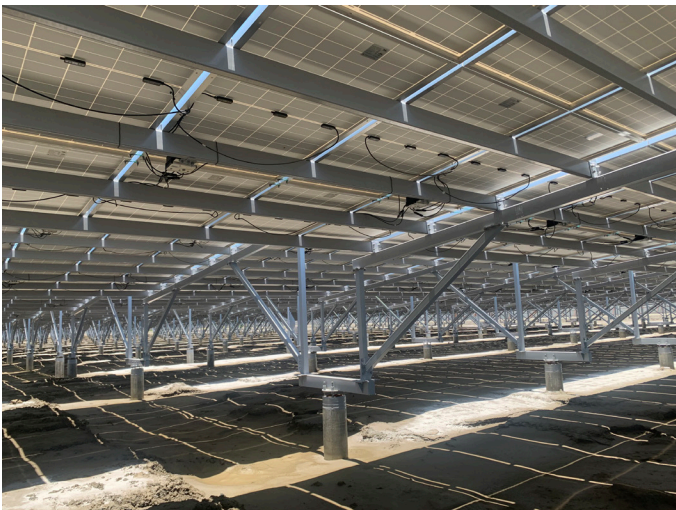
Fig 4: SolarEdge Power Optimizers connected to PV modules enable optimized energy output of the system
